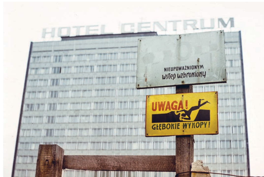
Warning! Deep excavation
